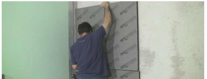
**5** When all panels are fixed seal the panel joints with the Stik tape
