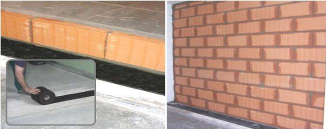
**2** Apply in the first wall a layer of row mortar of about 1 cm thickness
