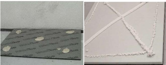
**4** Apply the panel on the wall by forcing with homogeneous pressure
